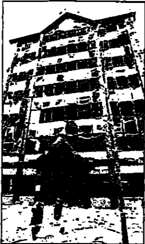
South Quay: damage was put at £150 million
